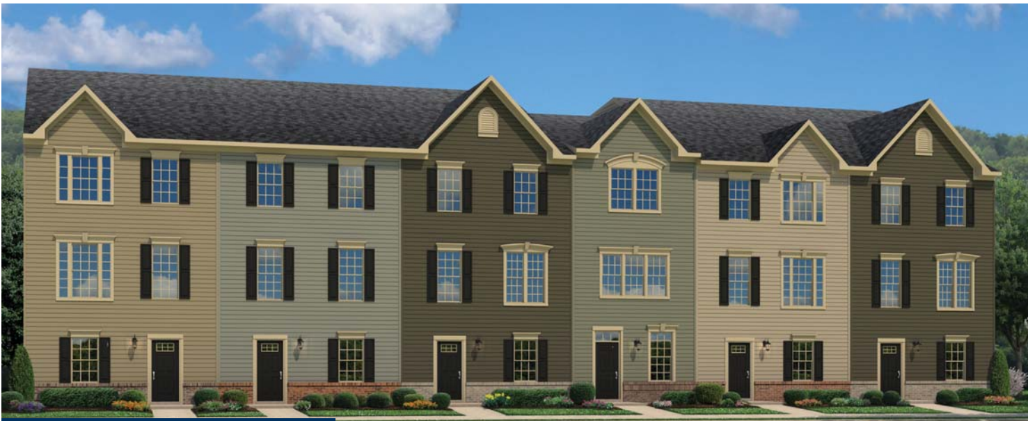
BASEMENT LEVEL ENTRY W/ REAR GARAGE
