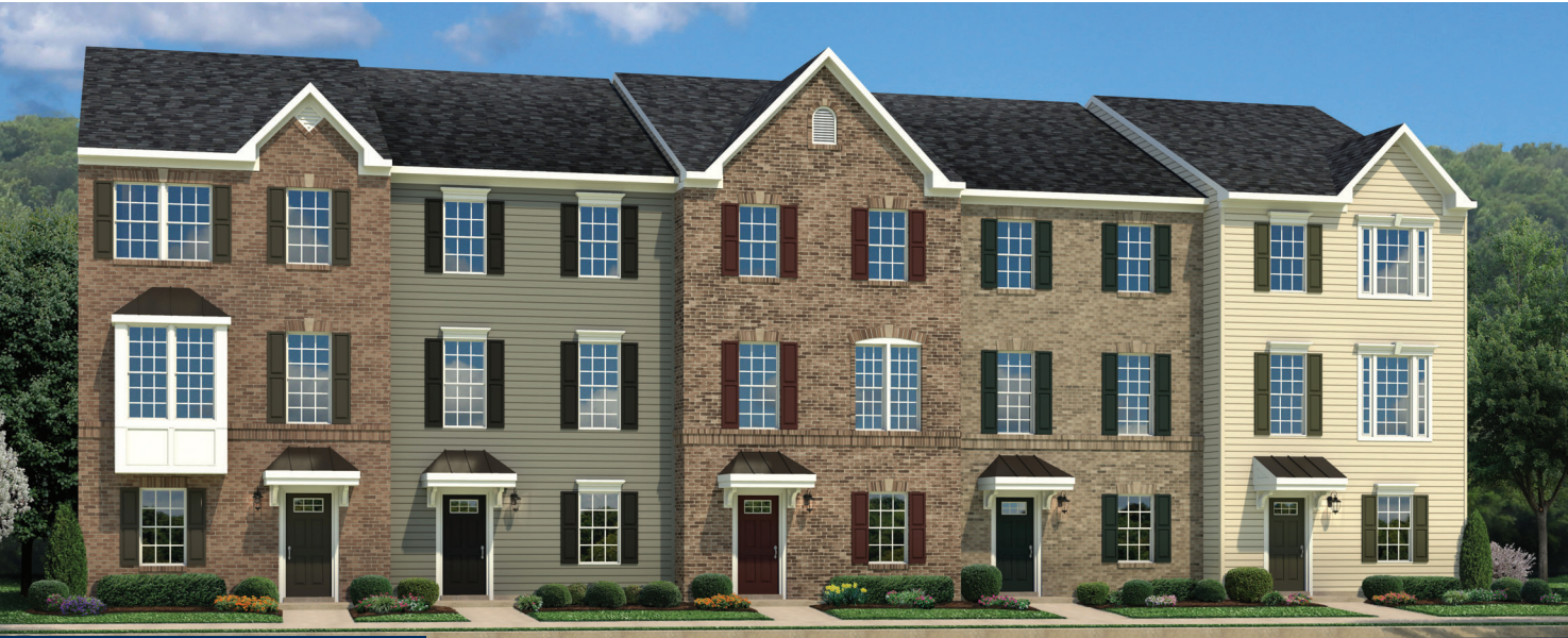
LOWER LEVEL ENTRY
