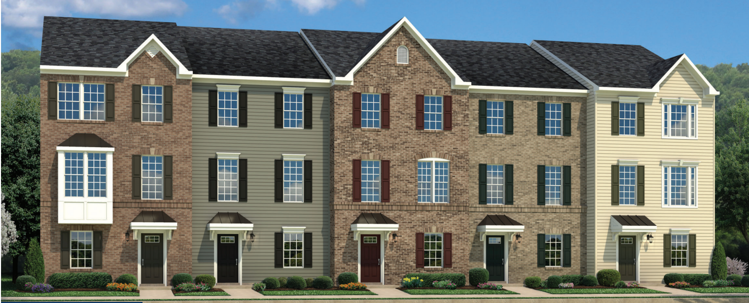
LOWER LEVEL ENTRY
