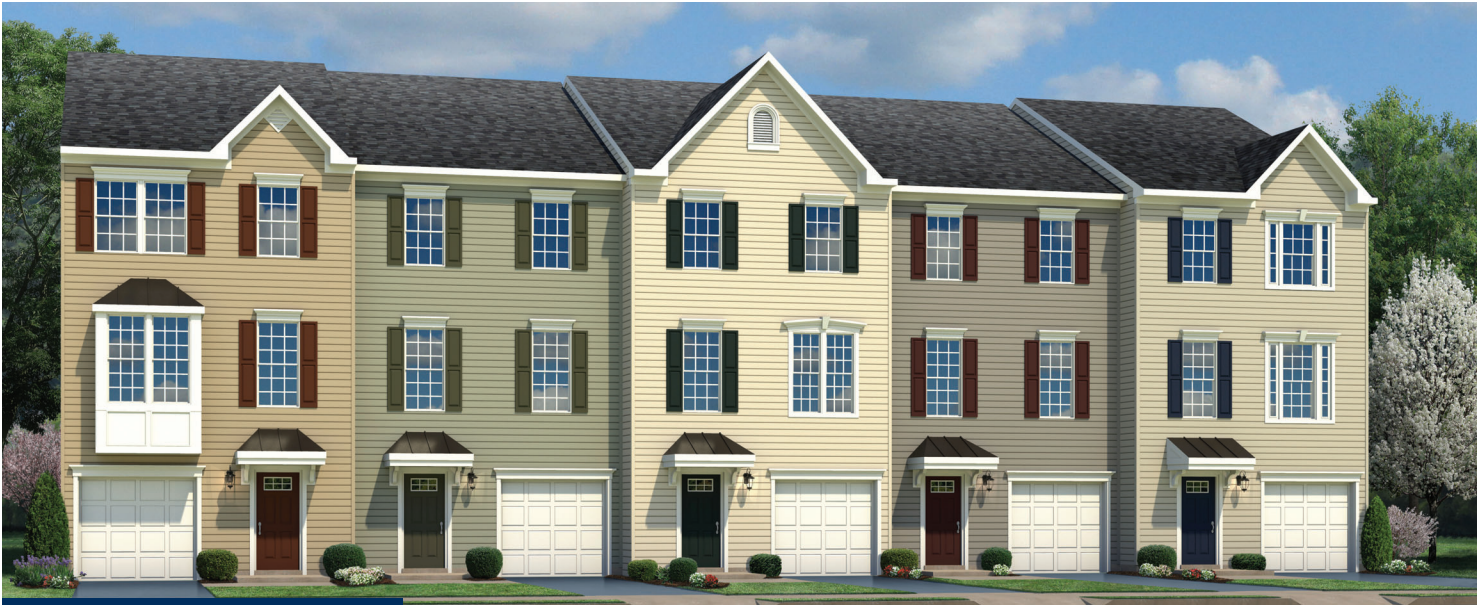
BASEMENT LEVEL ENTRY
